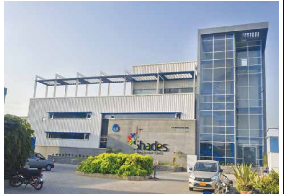
A view of the Masterbatches facility at ICI Pakistan Limited's West Wharf premises, Karachi.
