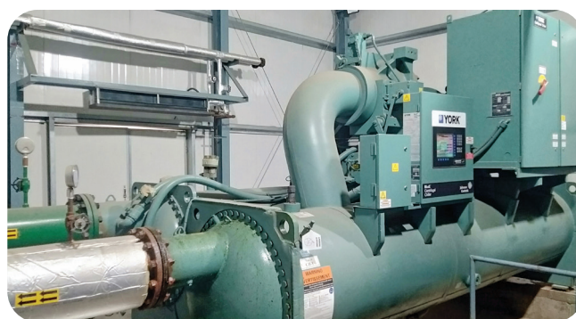
VFD-driven 650 USRT chiller at the Polyester plant, Sheikhpura.
