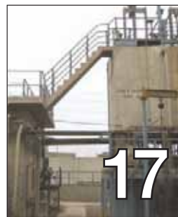
Effluent Treatment Plant
