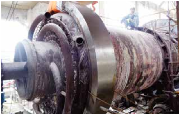
The Soda Ash team successfully replaced the calciner ring at the Soda Ash plant, improving efficiency.
