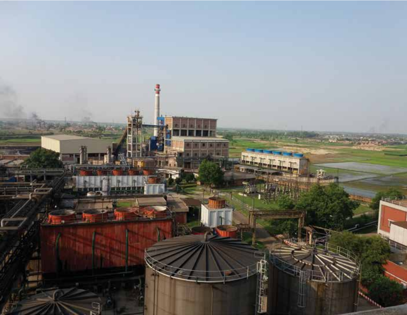
A view of Polyester plant in full swing
