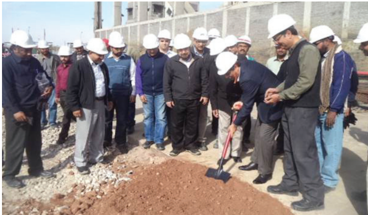
March 13, 2015, marked the start of the construction work.
