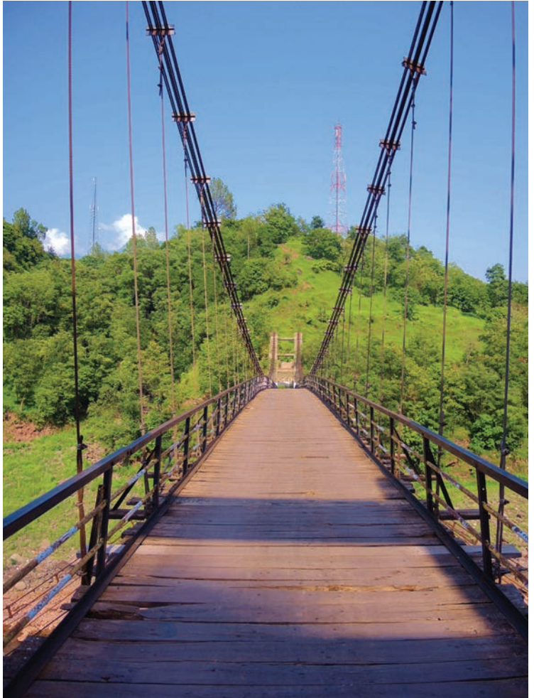
Bridge near Chakoti Sector, Kashmir.
