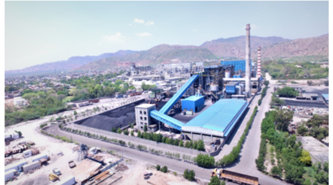
Soda Ash Plant, Khewra
