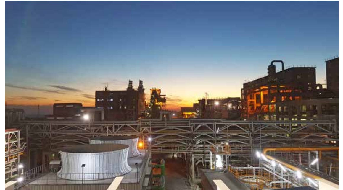
An evening view of the Soda Ash plant at Khewra
