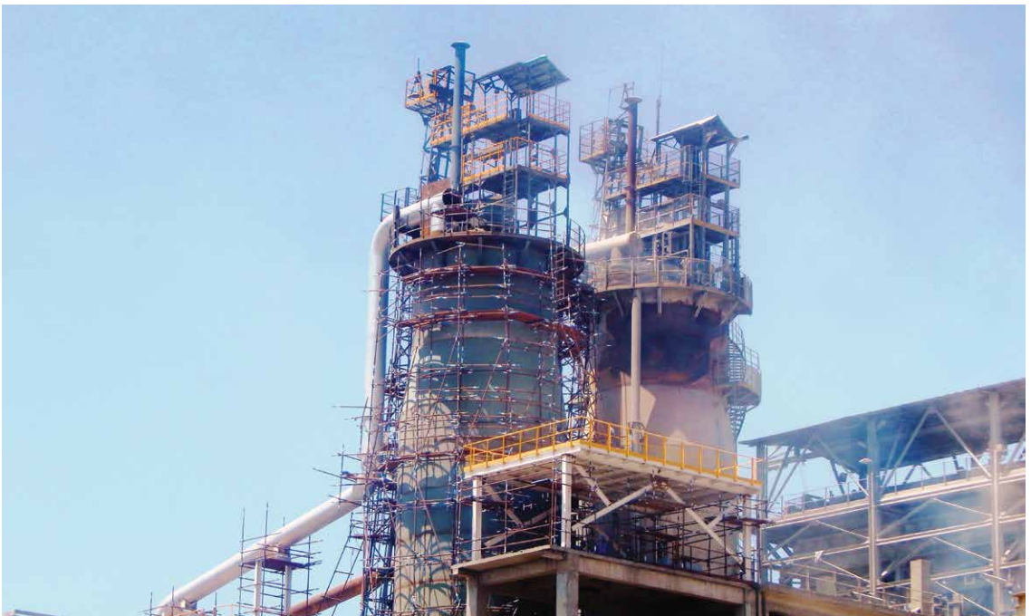
The new Kiln-8 during construction.
