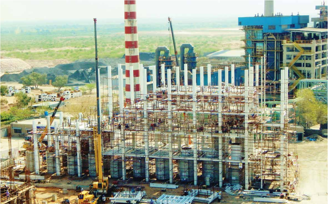
Constructing the building's steel structure safely and effectively.
