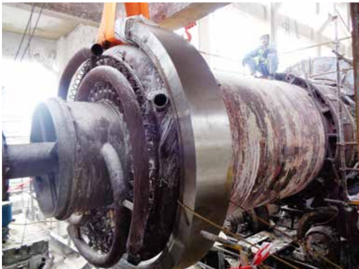
The new tyre is moved into position.
