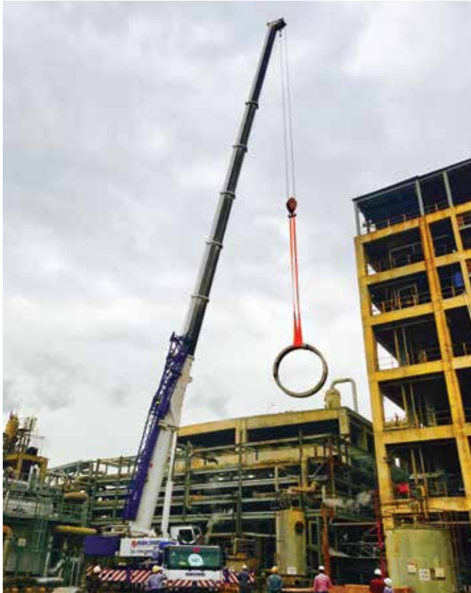
Replacing the Calciner ring.
