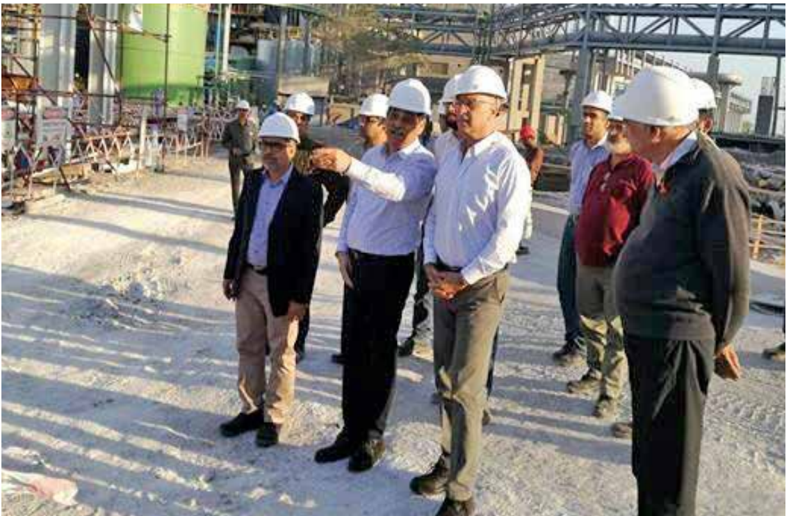
Asif Jooma (CE) visits the construction site with Suhail A Khan (VP Polyester and Soda Ash Businesses) and team members.
