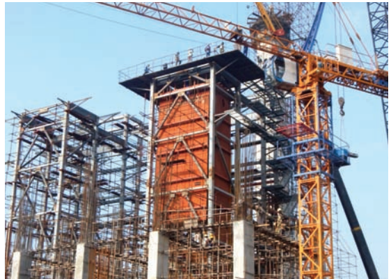
Power generation project under construction at Polyester.
