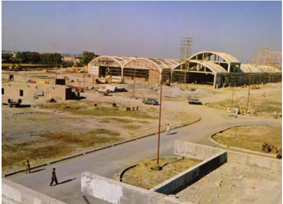
Polyester Plant under construction.
