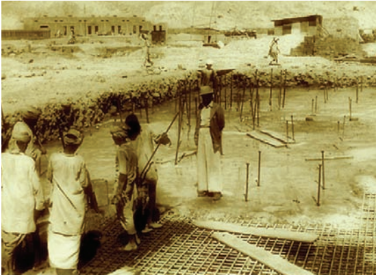
Laying foundations at Khewra.
