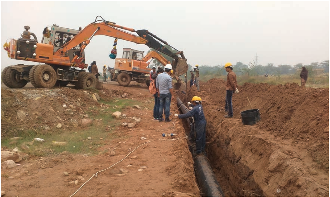
Excavation for the water pipeline in progress
