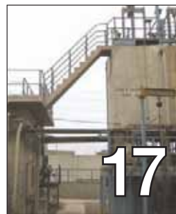
Effluent Treatment Plant
